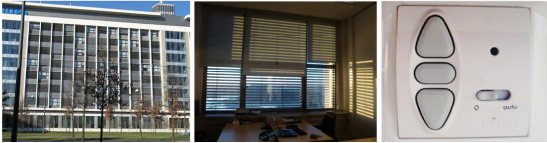
Fig. 1: Office building at the High Tech Campus (left), 2-person office with internal shades and external blinds (center), blinds controller in the office (right)
